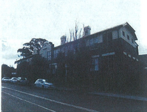
Photo 11: Auburn Public School Beatrice Street frontage
