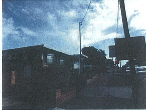
Photo 4: Southern side of Beatrice St looking west
