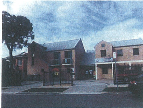
Photo 15: Community centre to east on Susan St
